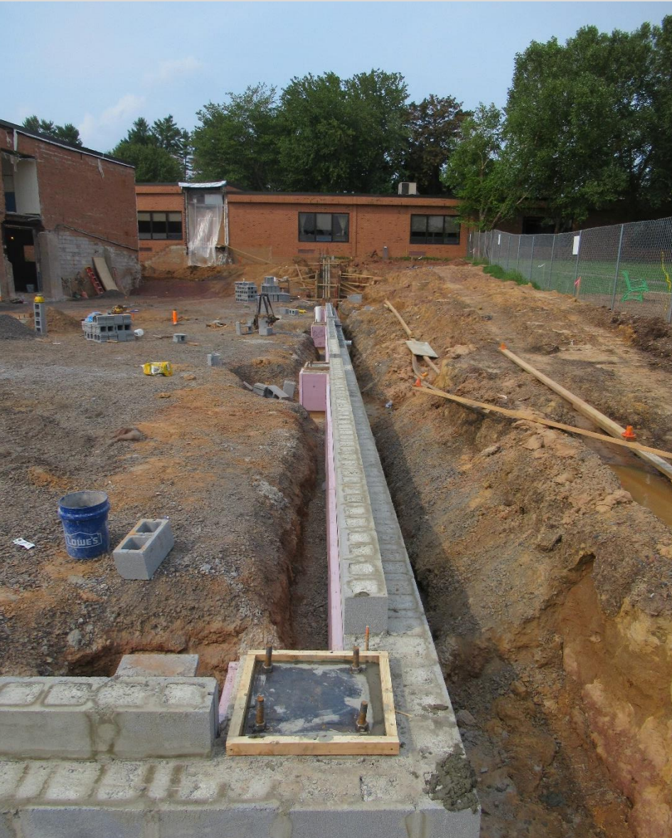
New Classroom Wing – Footings, Foundation Walls and Piers
